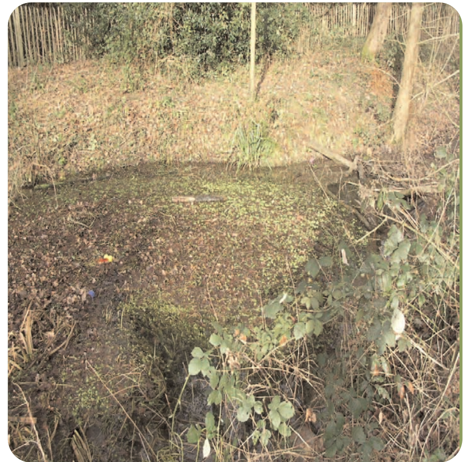
Pond requiring restoration by removal of rubbish and vegetation
