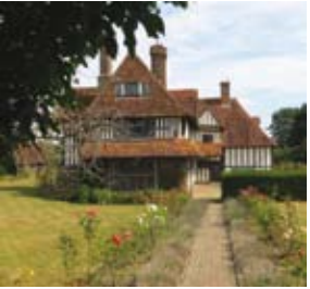
Timber Framed House
